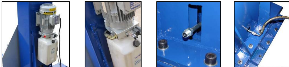
Fig. 7-A, B, C, D pump & hose
